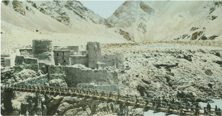
Khaltse Bridge over the Indus River, as it existed in 1948 (photo credit wikipedia.org)
