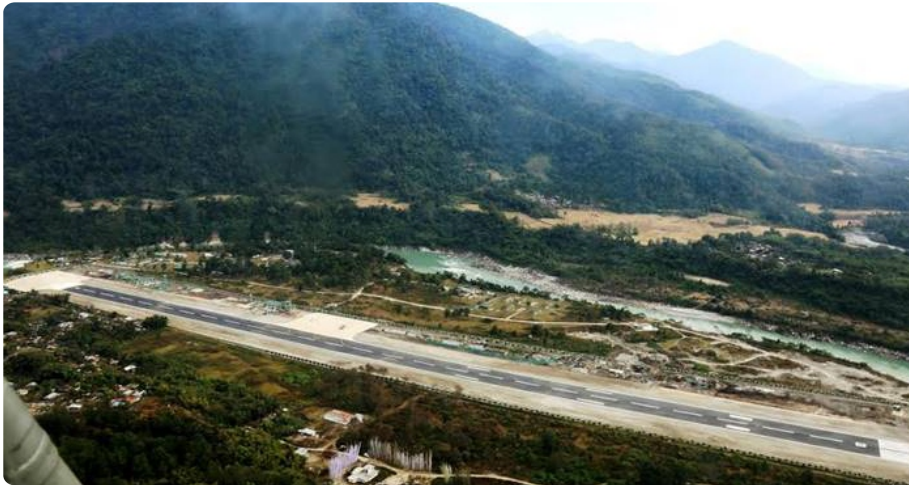
Advanced Landing Ground in Tuting (Photo: @CMPemaKhandu)
