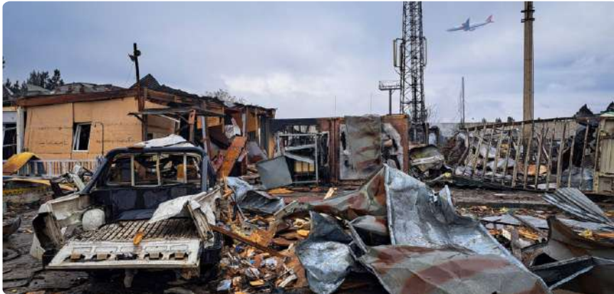
Damages near Kabul Airport, after Pakistani airstrikes
