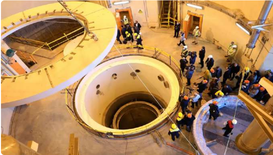
The Arak heavy water nuclear reactor in Iran, specifically the calandria (core) area. In June 2025 Israel reportedly conducted an attack on this reactor facility (Credit Radio Free Europe Radio Liberty)
