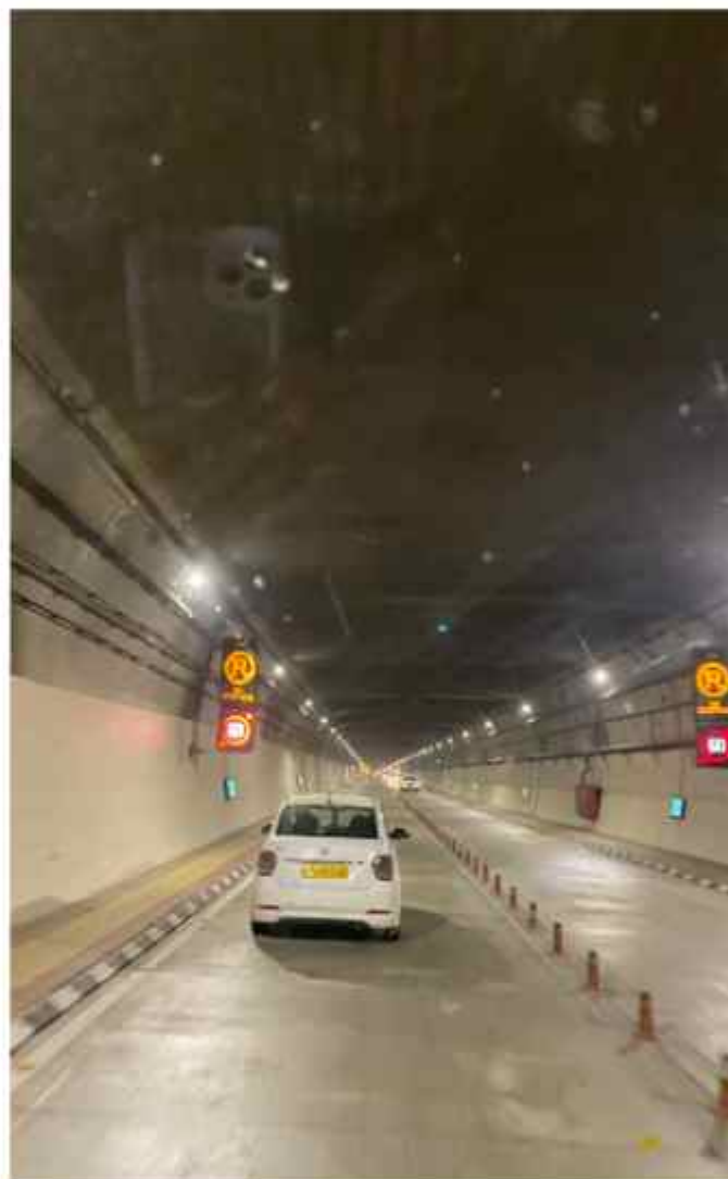
Atal Tunnel (Rohang Tunnel), 07 September, 2022 (credit common.wikimedia.org)
