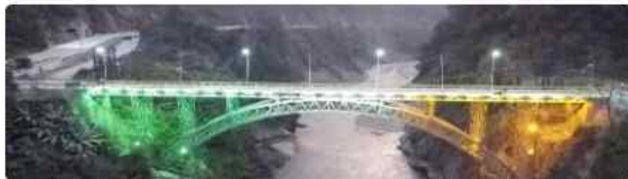
Siyom bridge in Arunachal Pradesh is the first signature arch bridge made by BRO
