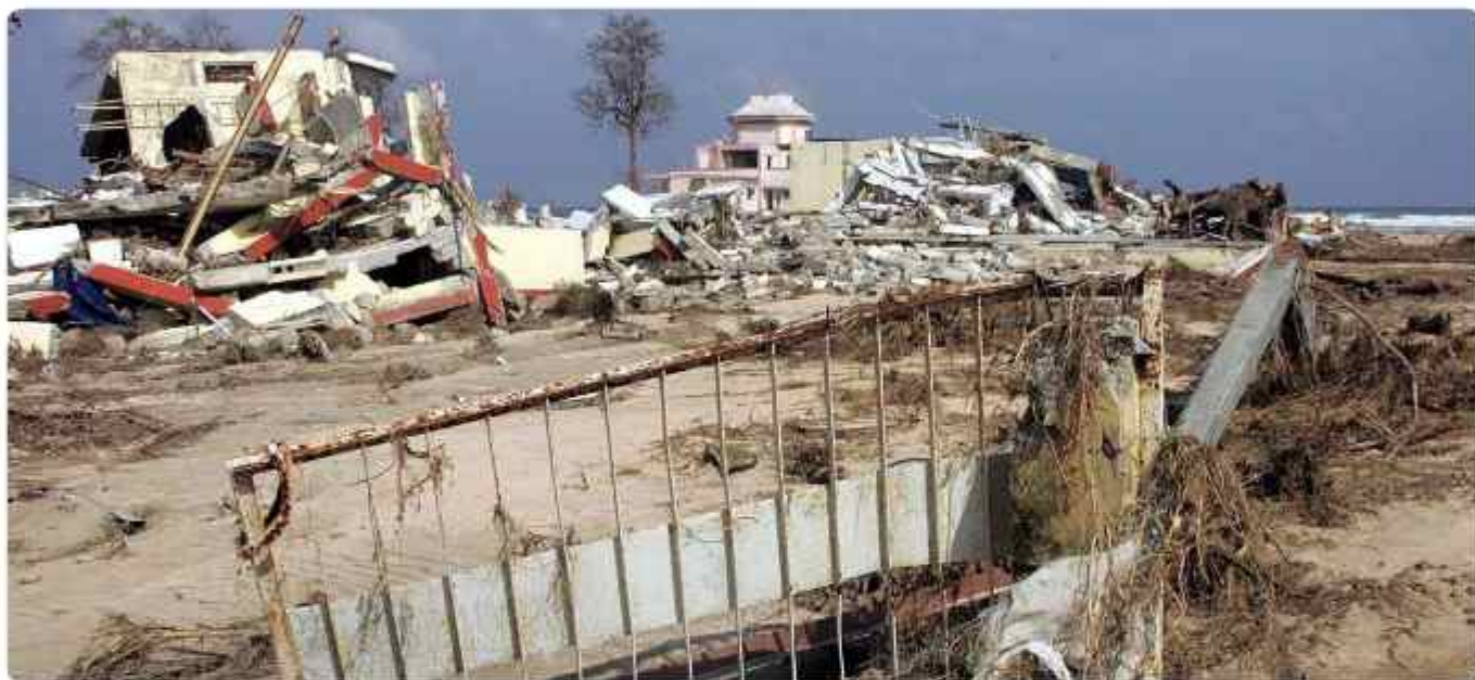
Damaged Indian Air Force buildings on Car Nicobar island after the tsunami hit on December 26, 2004 (Photograph: Jayanta Shaw SD/SM/Reuters)
